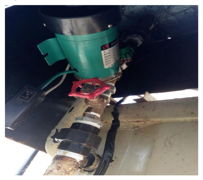
The pump is a 0.5HP is fitted on the side of the dryer container. The pump sucks warm water from the water pipes of the water exchangers to the water tanks. This sucking moves the water within the whole system.
