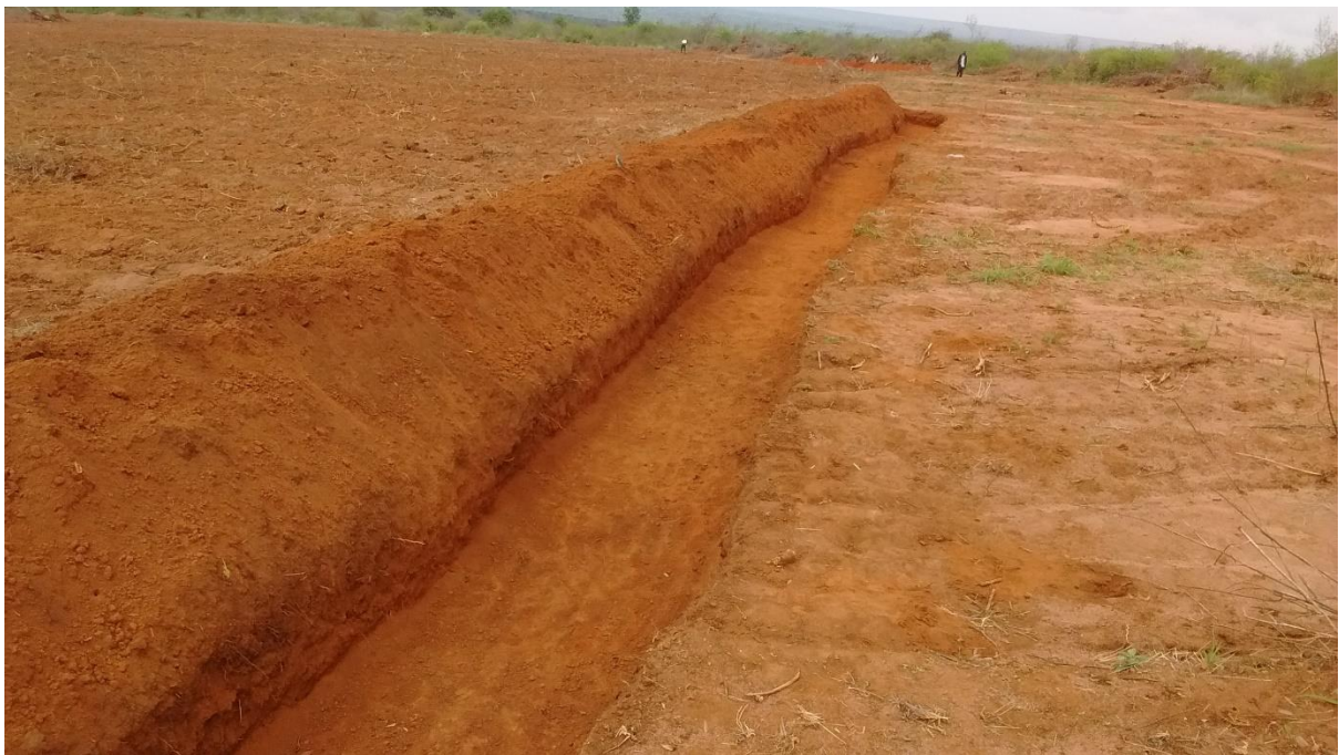
Trench for rainwater catchment and soil conservation
