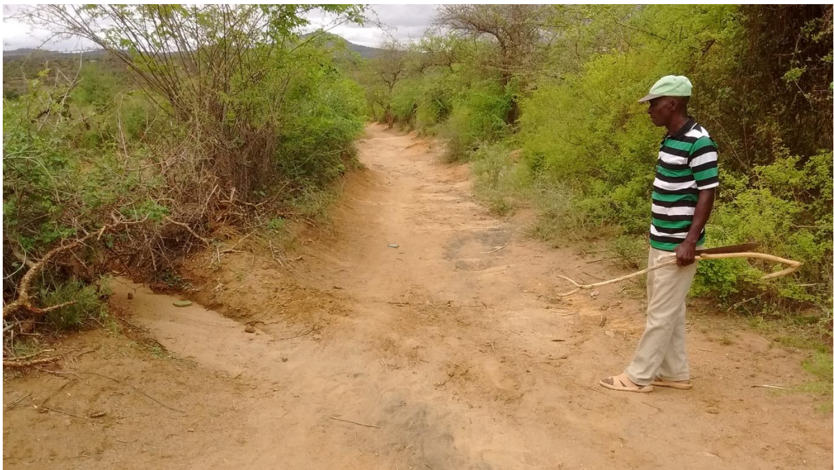
Diverting and harvesting runoff (flood) water from roads into farms
