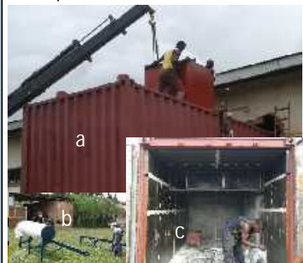
Dryer being built by local artisans: a) Installing the dryer at the project site; b) Assembling the solar system; c) working on the inside
